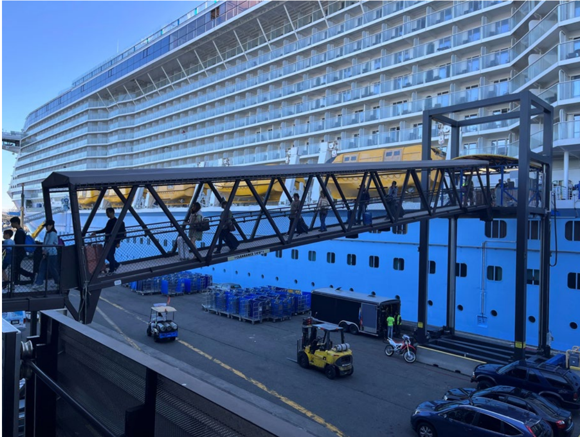
Existing passenger secondary gangway at Pier 91 East cruise berth
